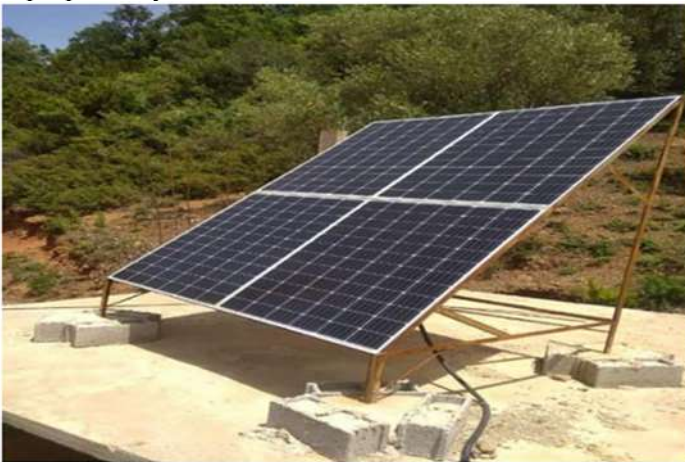
Fig.8 PV installation system
