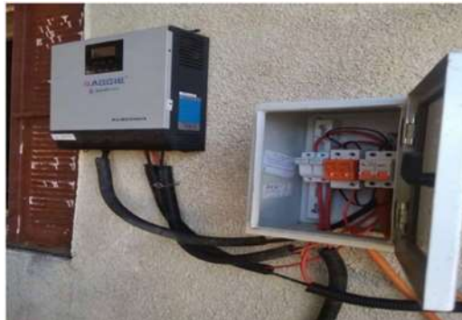
Fig.4 MPPT converter
