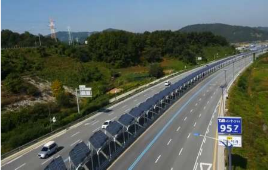
Figure 4. Application of Solar Panel Bicycle Path in South Korea
