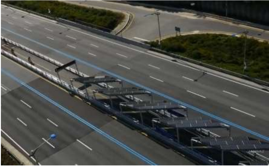
Figure 8. Proposed Solar Panel Installation on the Median Strip and Bicycle Path Below the Panels.
