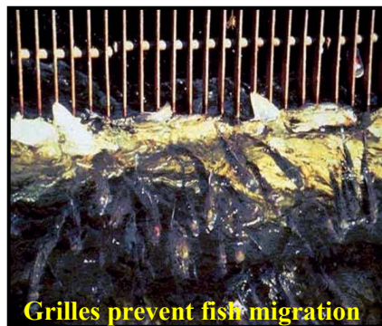
Figure 3. Fish passages in turbines, grilles prevent fish migration (Berkun et al., 2008:44).
