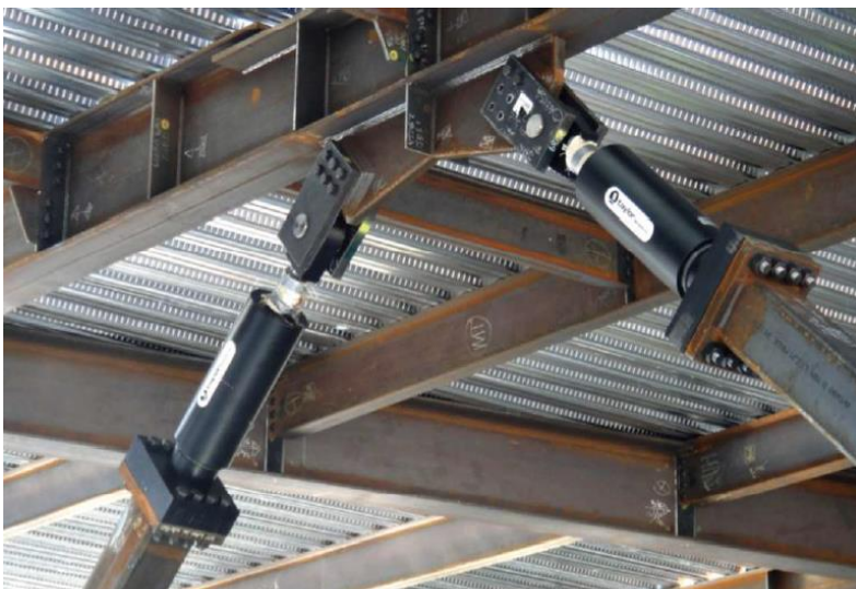
Figure 5. Fluid viscous damper appearance in structure
