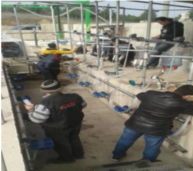
Figure 2: Installation of a milking parlor (Aydin, 2016)
