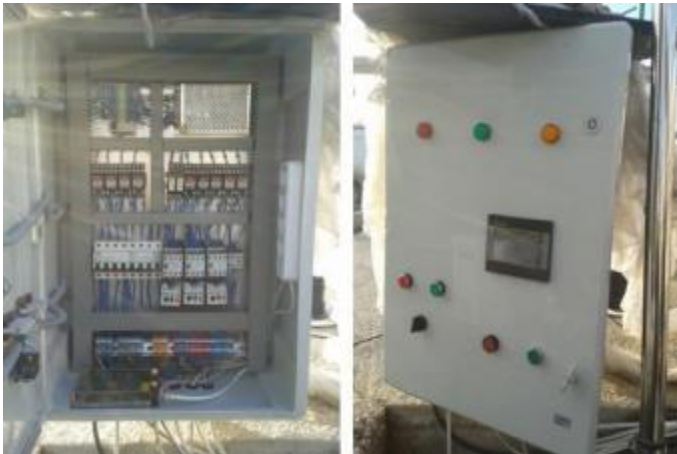
Figure 8: PLC controlled milking parlor panel (Aydin, 2016)
