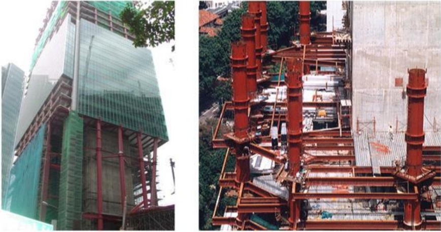
Figure 5: Use of concrete-filled steel tube in high-rise buildings (Liew et al., 2016)
