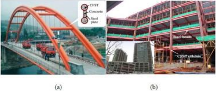
Figure 5: Use of concrete-filled steel tube in high-rise buildings (Liew et al., 2016)
