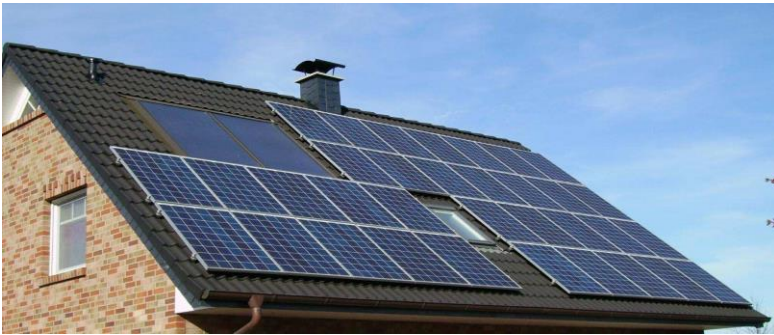
Figure 3. A photovoltaic solar energy system used in a residential building [13]
