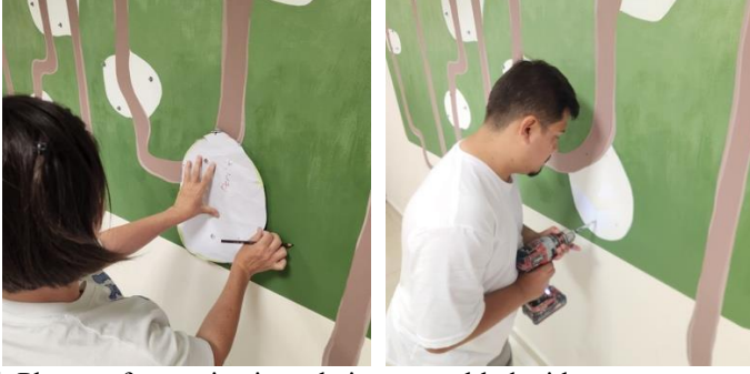
Figure 6: Photos of ceramic pieces being assembled with smart screws (Personal Archive, 2025).
